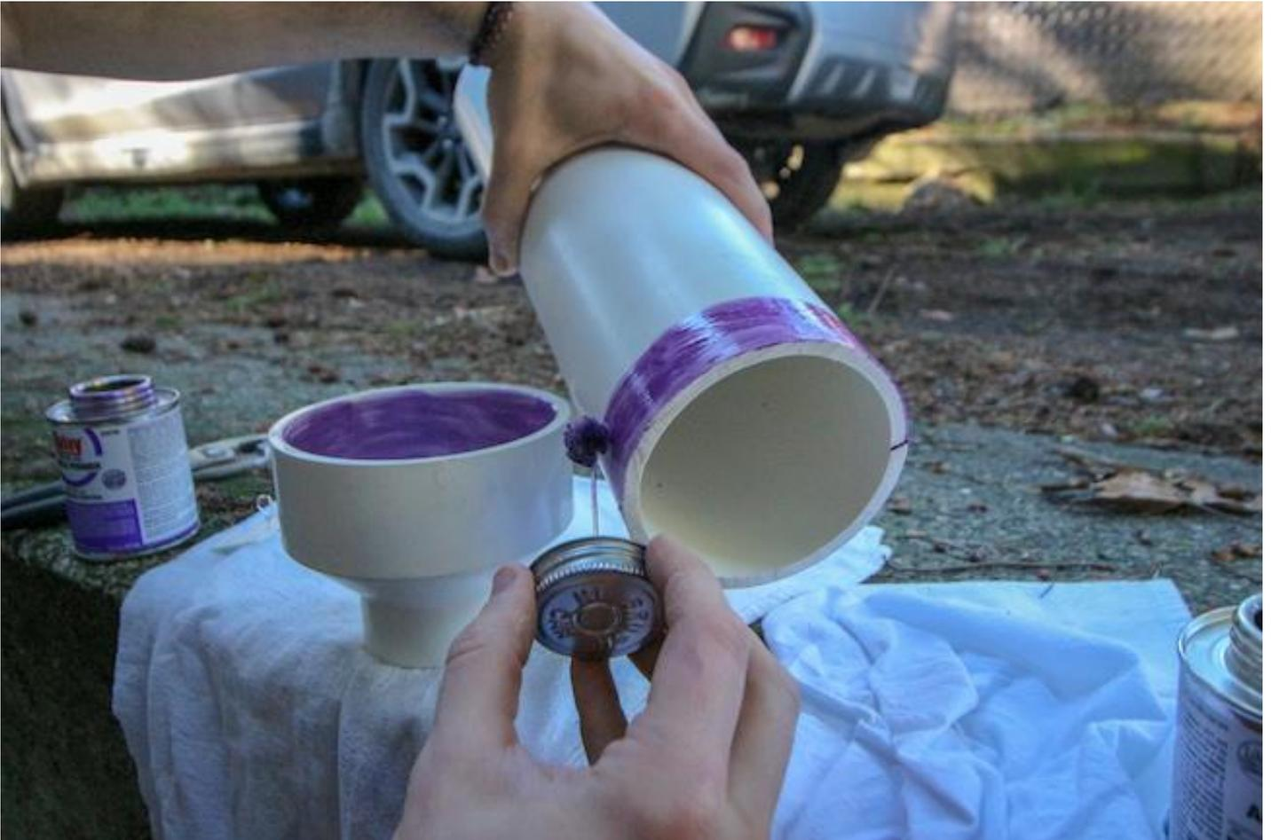
To glue PVC together, start by priming both pieces with PVC primer (purple in the photos), let it dry for 10 seconds, and then apply PVC cement. Once both parts are primed and glued, push them together, give them a quarter turn, and hold for 30 seconds until set.
