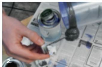
**2. Brush on a thick coat of PVC solvent, first to the end of the pipe, and then to the fitting socket. Leave no bare spots.**
