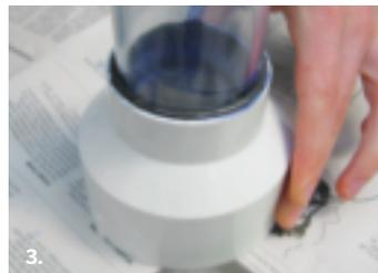
**3. Immediately join the pipe and the fitting socket, pushing the pipe to its full depth and making sure it's seated squarely with a slight twist. If you've used enough solvent cement, you should see a small, continuous ooze of cement around the fitting. Once joined, you can't reposition the pipes or otherwise fix errors. If you accidentally put the wrong fitting on a pipe, you need to trim it off and start over.**
