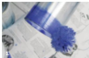
**1. Clean the weld surfaces with PVC primer. Apply the primer with a dauber or brush (usually inside the cap). The primer cleans and softens the PVC and allows the cement to penetrate the surface.**
