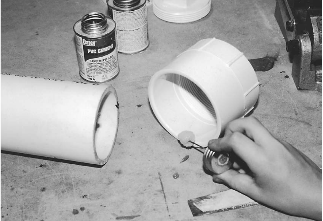
2.3 Applying the PVC cement
